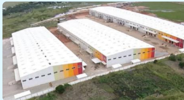
Location: Maputo, Mozambique Status: Nearing Completion Size of Park: 290,000m 2 Leaseable Area: 32,000m 2
